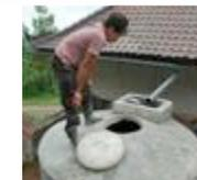
**precast ferrocement septic tank**
